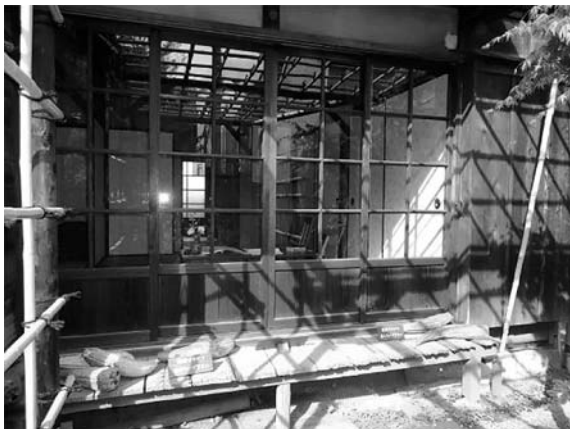
Photograph 8 The recuperation room that looked from garden
